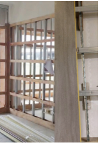
Steel Frame + Studs Base Board Not Required
